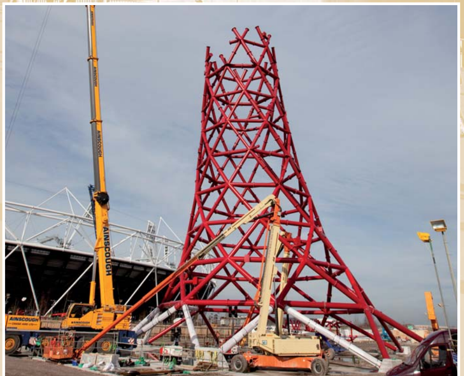
Courtesy of ArcelorMittal
