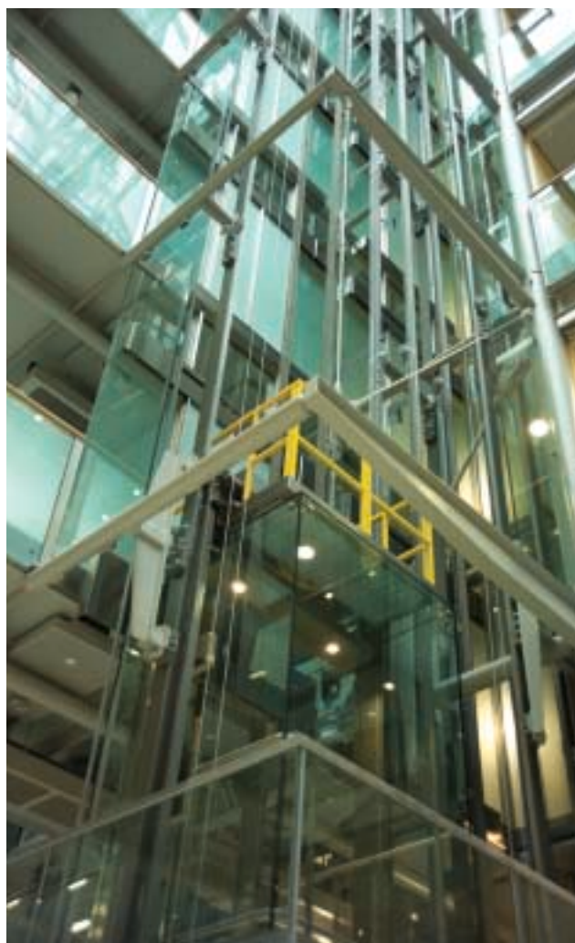
Kone lift at the new Wellcome Trust Gibbs Building, Euston Road, London
